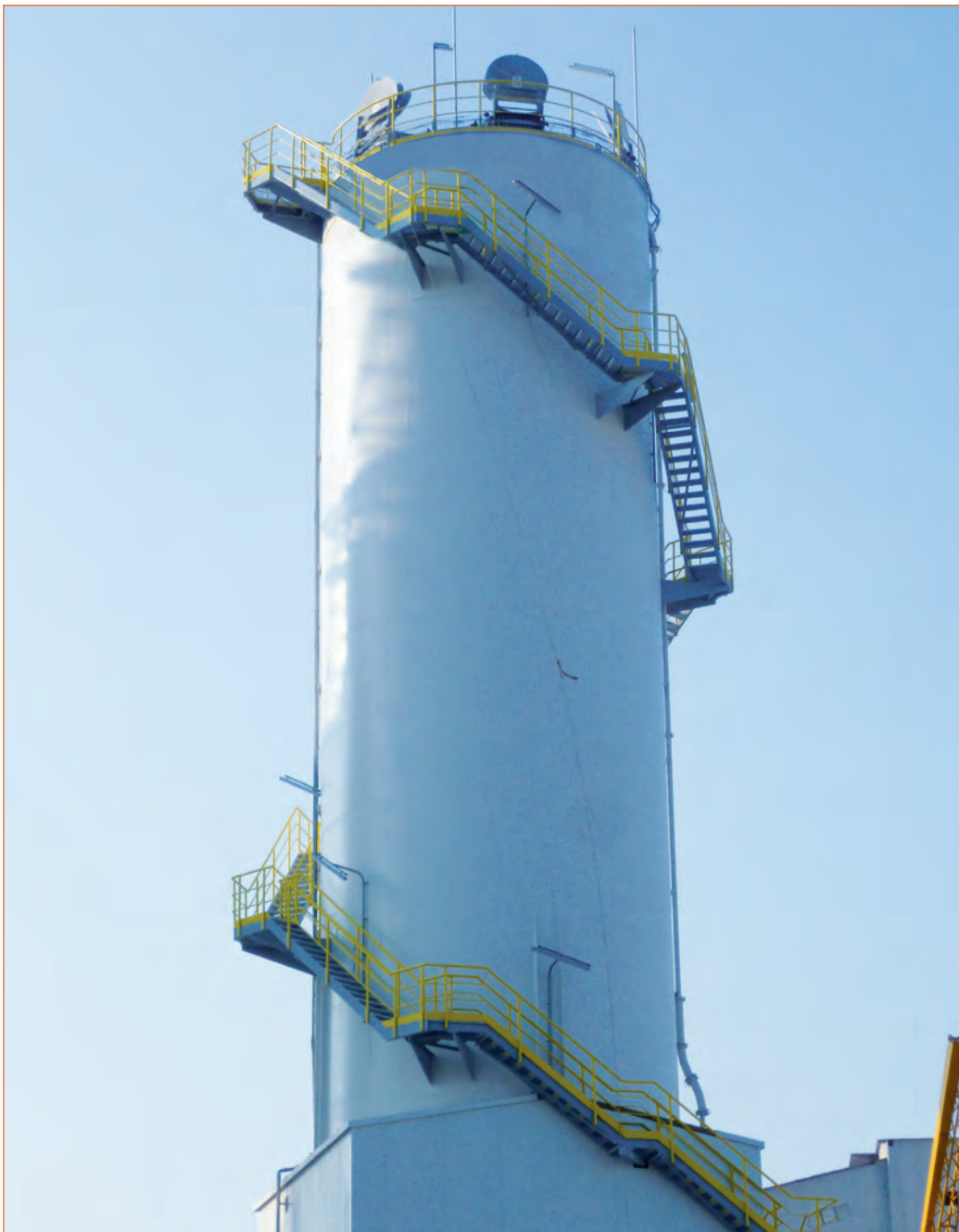
1.100m 3 silo for brown coal dust for the firing of a lime shaft kiln
