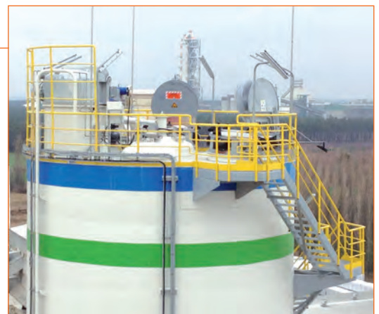
Flat roof design of a typical coal dust silo
