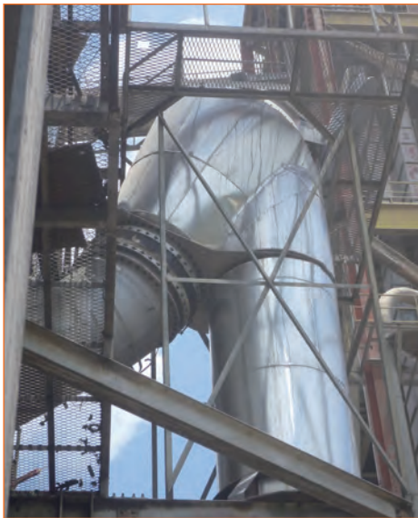
Mill-to-filter duct with propagation mitigation 1+2
