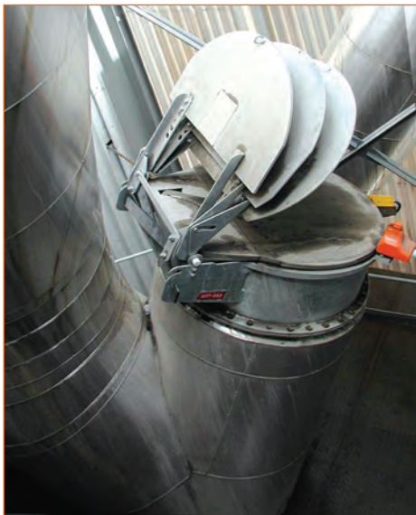
Mill-to-filter duct with propagation mitigation 1+2
